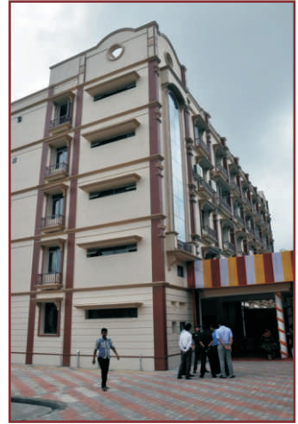
New building of Area Accounts Office, Kolkata, LAO(A) (B) (C) (D) & RAO (MES), Kolkata
